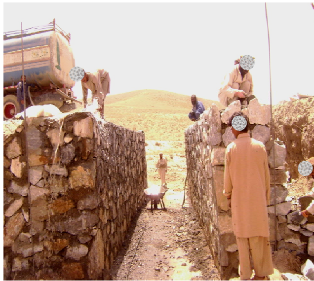
Site Photo 9: The wing walls of a stone masonry foundation for one of the 29 box culverts required by the project design plan. Of note are workers properly curing the cement mortar in the upper left hand corner of the photograph in order to allow it to develop its bonding strength. (Photo provided by Kapisa PRT)
