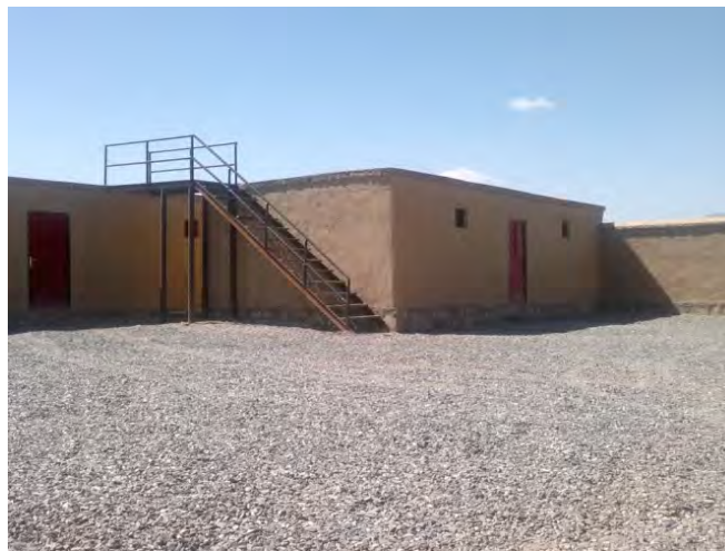
Photo 1 - Example of Completed Construction
