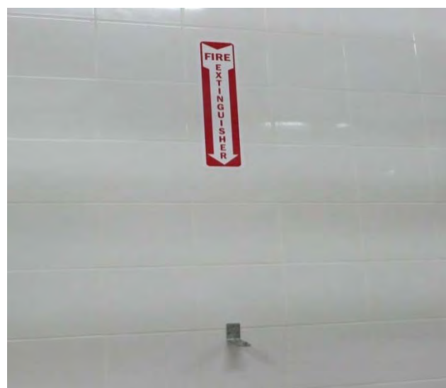
Photo 3 - Missing Fire Extinguisher in Barrack Building
