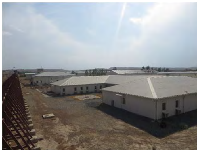
Photo 1 - Newly Constructed Buildings on the ANP Women's Compound
