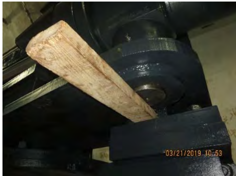
Photo 2 - Lumber Supporting the Emergency Closure Valve Pins
