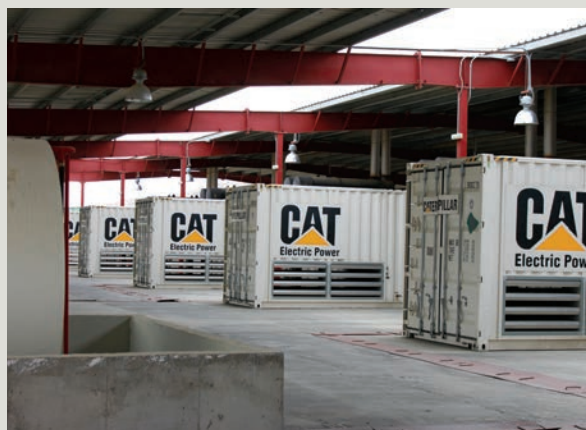
Diesel generators are used to provide electricity until NEPS and SEPS can be expanded and connected. (SIGAR photo by Steven Mocsary)
