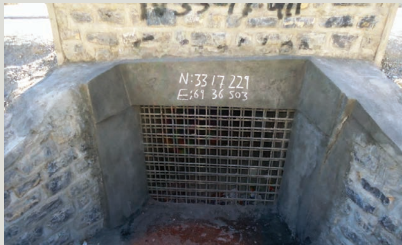
Culvert-denial systems like this grid of steel rods prevent insurgents from easily placing explosives beneath roads. (SIGAR photo)
