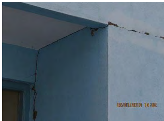
Photo 16 - Exterior Crack in 8 Classroom School
