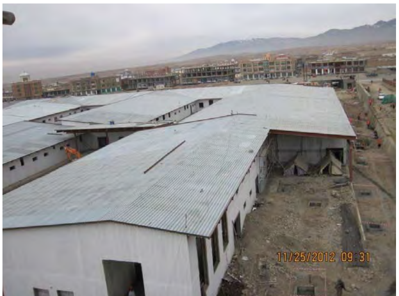
SIGAR photo of Gardez hospital under construction, November 2012
