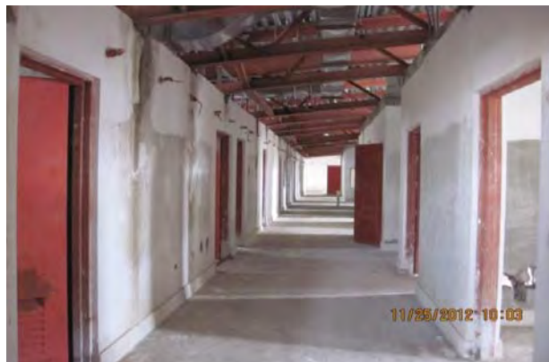
SIGAR photo of Gardez hospital under construction, November 2012
