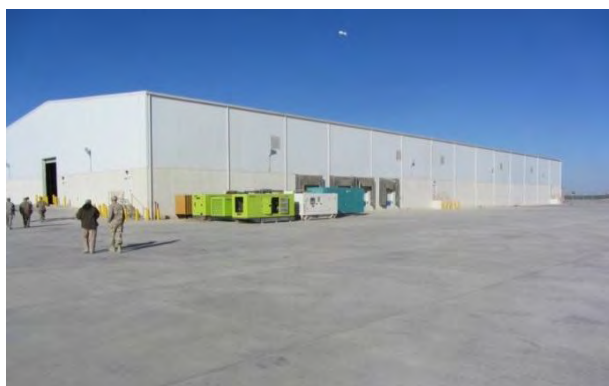
Photo 1 - Warehouse Building at KAF
