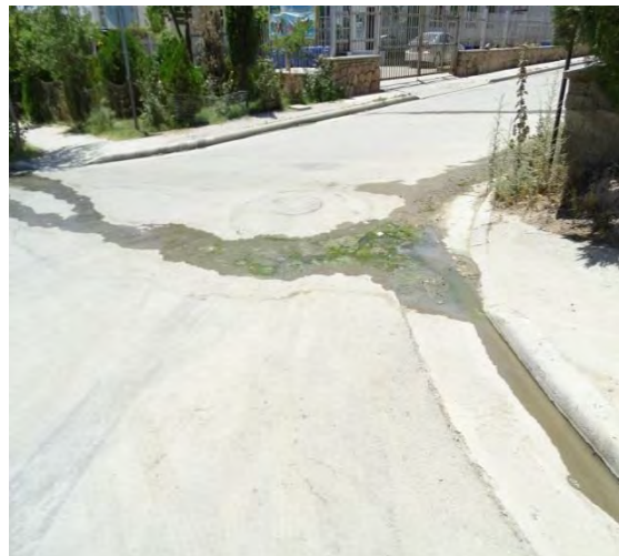
Photo 3 – Untreated Factory Water Flowing into the Park's Streets
