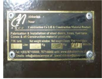
Photo 8 - Noncertified Fire Door Installed in Gulbahar Substation
