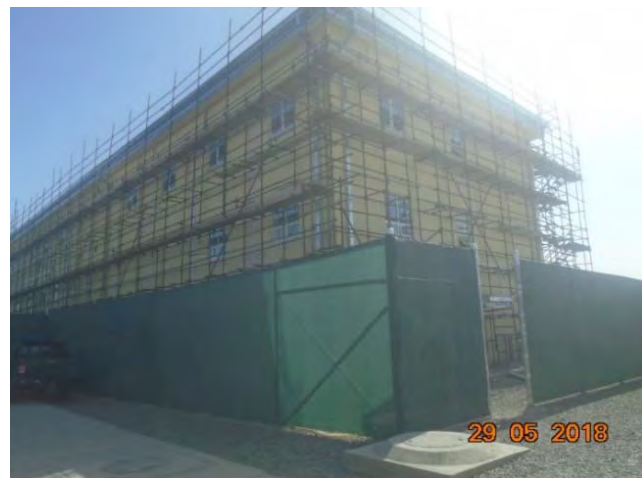
Photo 1 - Multi-purpose Building Not Ready for Occupancy
