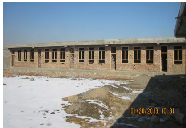
Photo 1 - New Classroom Building under Construction
