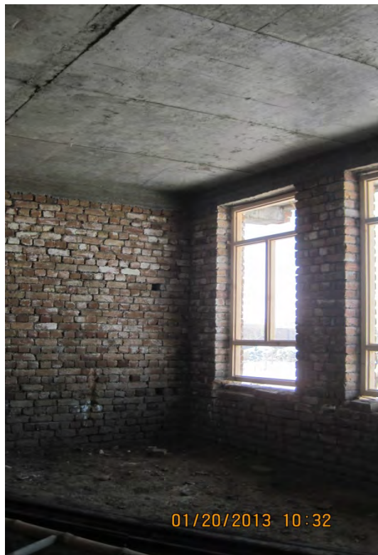
Photo 2 - New Classroom Construction with Brick Walls and Concrete Ceiling/Roof
