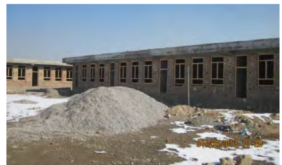
Two 5-classroom buildings under construction instead of single 10-classroom building
