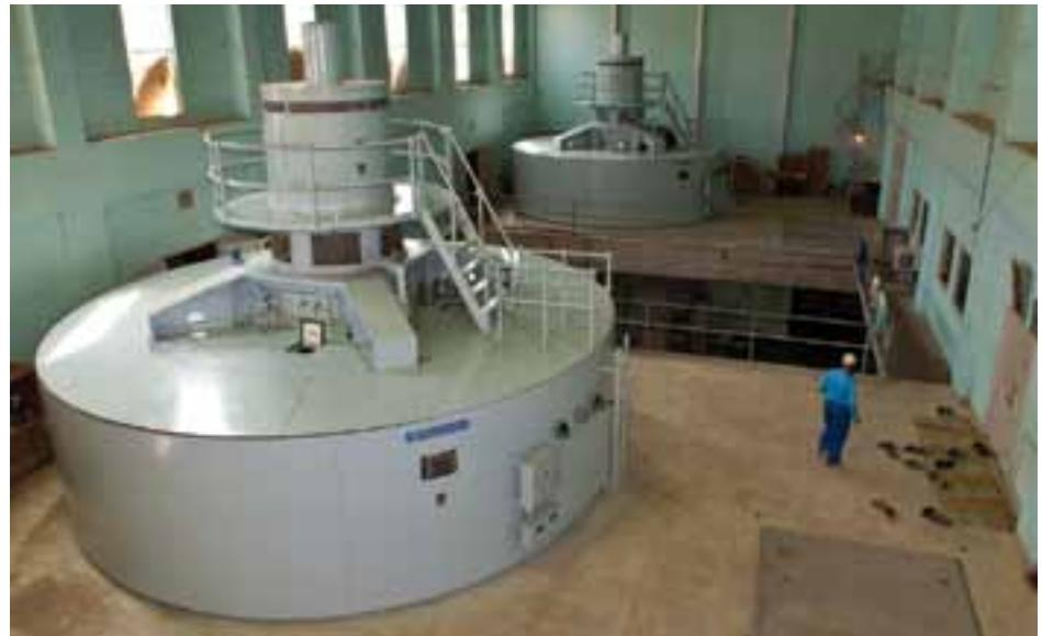
**Two hydroelectric turbines** at the Kajaki power plant produce 16.5 megawatts of electricity. Since 2009, plans to install a third turbine have been delayed by a lack of security. This quarter, U.S. Marines cleared the road to Kajaki, allowing the first convoy carrying equipment to reach the dam and return safely. Credit: U.S. Navy photo, MC Jonathan David Chandler.
