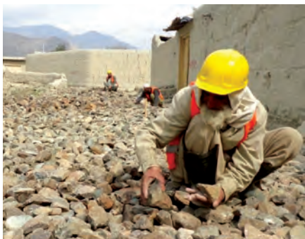
The Khani Baba street network repair project aims to rehabilitate 800 meters of village streets and drainage trenches to build confidence in the local government. (CCI photo)
