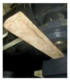
**A plank supports** emergency-closure valve pins in the Kajaki Dam Irrigation Tunnel. (SIGAR photo)
