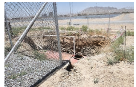
Temporary septic tank in use outside Pol-i-Charkhi Prison. (SIGAR photo)
