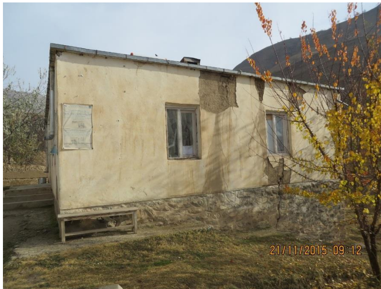
Photo 1 - Exterior of Health Facility 1987
