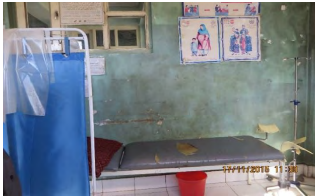
Photo 3 - Interior Room at Health Facility 406
