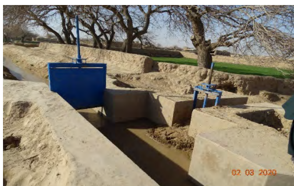
Photo 4 - Hasan Abad Canal
