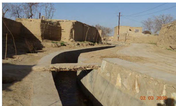
Photo 5 - Hasan Abad Canal
